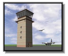
Construction Method: Load Bearing Masonry, w/ Structural Steel Cab
