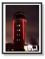
Construction Method: Structural Precast Concrete Shaft; Steel Frame Cab
